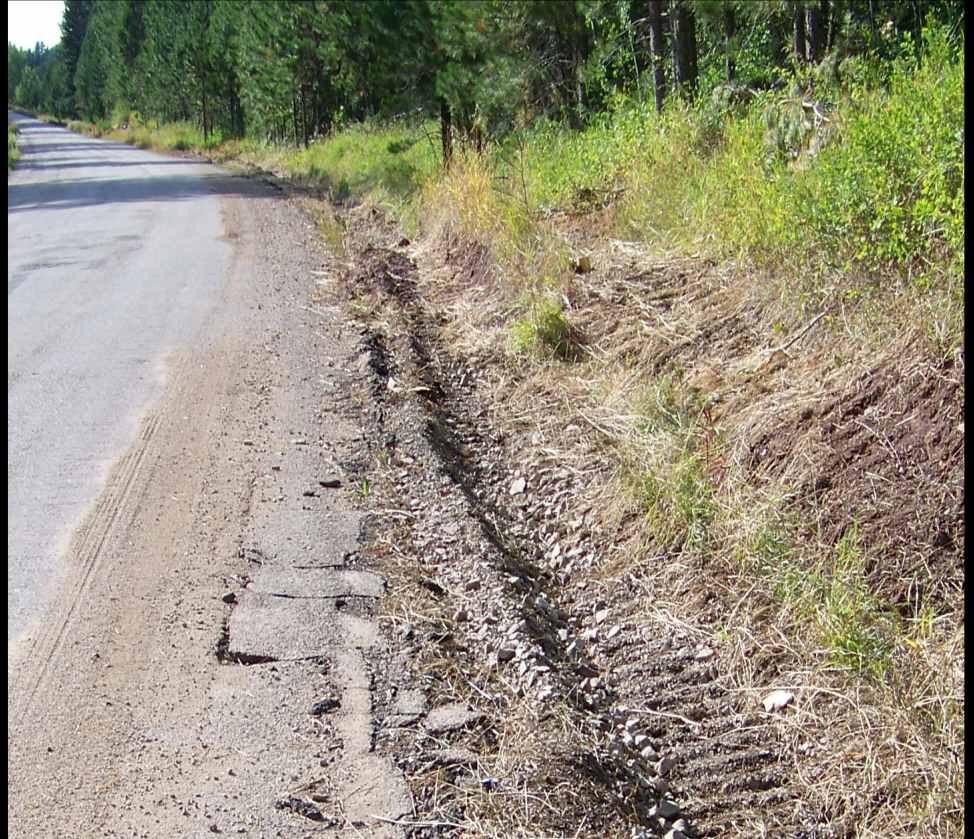
Fergus Electric Transmission Repair circa.(2008)
